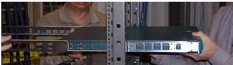
Figure 1-5: Sliding the Switch Into the Rack
