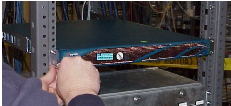
Figure 1-9: Secure the Switch Through the Front Posts
