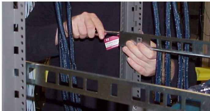
Figure 1-4: Secure Rack Brackets to Rack with Screws
